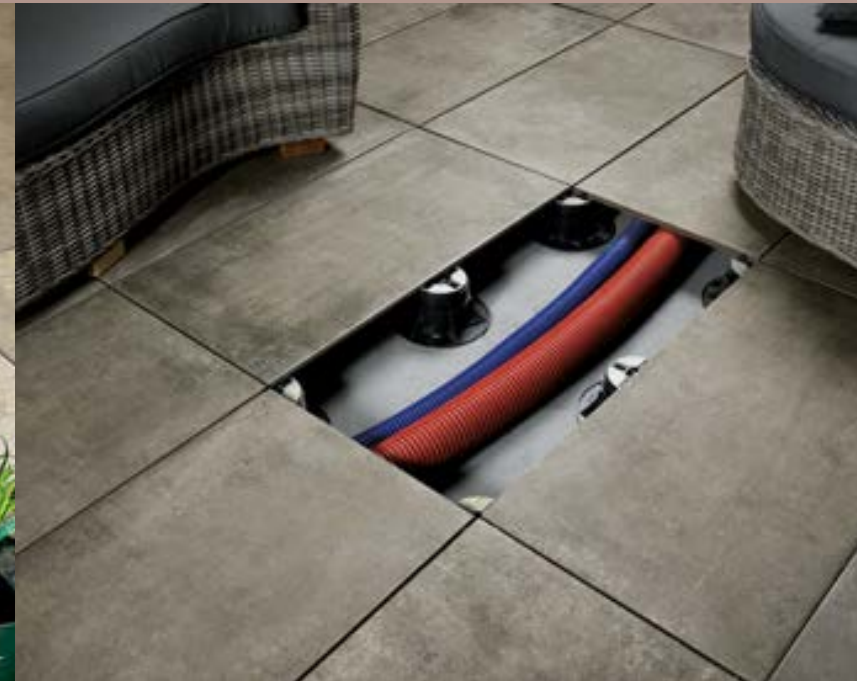
POSA SOPRAELEVATA RAISED LAYING
